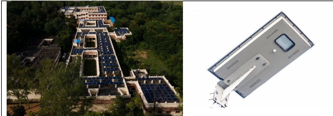
Roof top Solar Panels (Department of Forestry) 22°07'36.2"N 82°08'21.4"E
